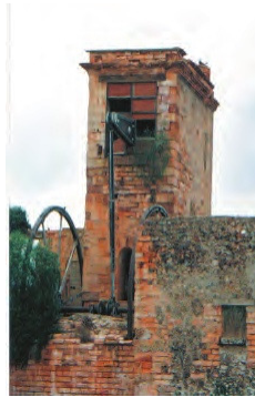
Figura 9. Bomba “Cornwall Engines”.
