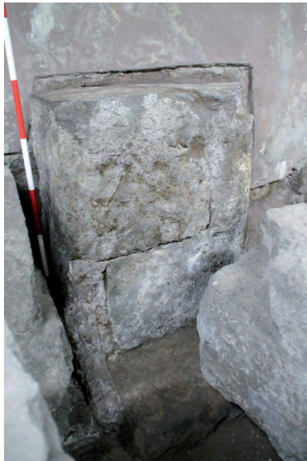
Figure 4. The first pillar of the oriental portico of the Area Sacra of Largo Argentina partially embedded in the modern masonry.
